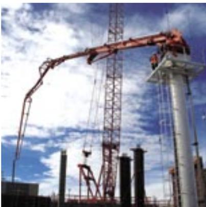
*A detachable boom option allows you to remove the placing boom for job-site versatility with a variety of mounting options including free-standing, form mounting or mast-mounting with floor frames.*
